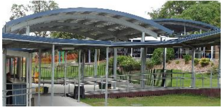
The two Preparatory Covered Areas
