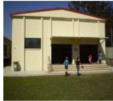
Activity Indoor General Purpose Building
